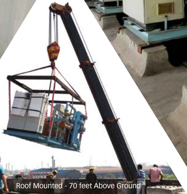
5 x 150 TR Roof Mounted at Tarapur
